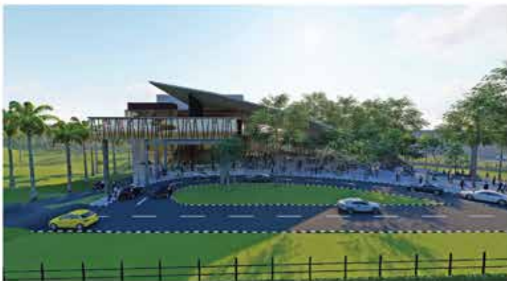
MULTI-PURPOSE CONFERENCE HALL
